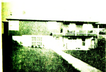
Newest project of Benton home missions—a parsonage built with all volunteer labor.
