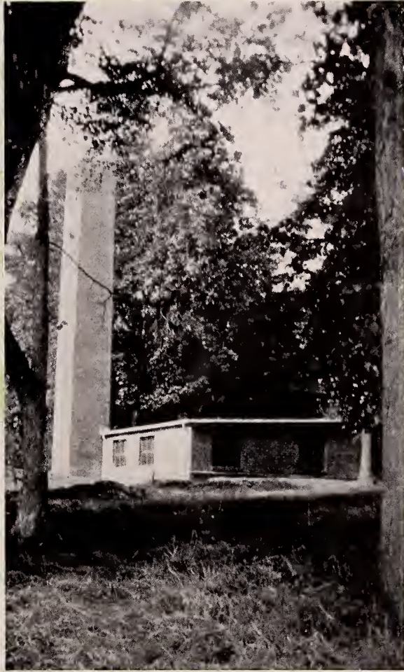
The Heating Plant
